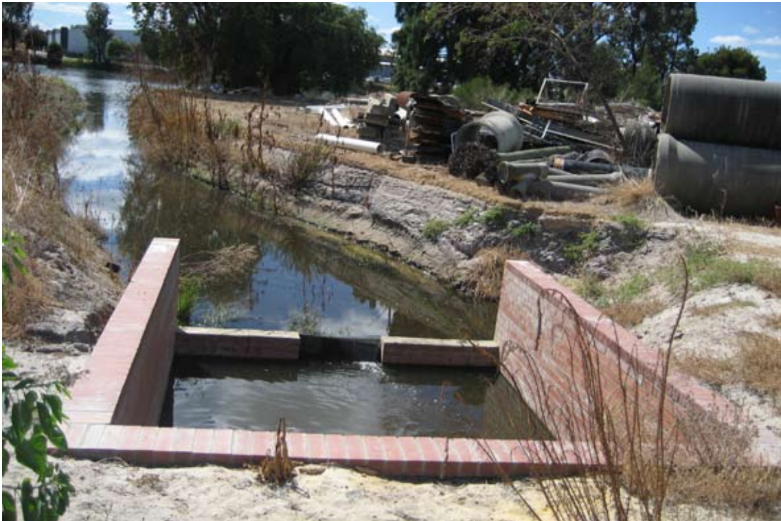
Mill Street Compensating Basin Outlet 2007
