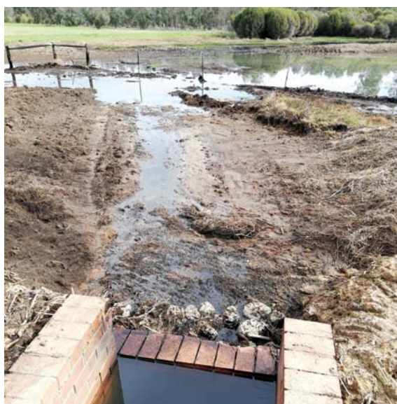
Drainage culvert from Roe Highway after earthworks and removal of couch
