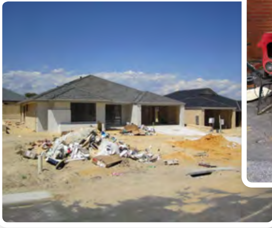
Builders sand is blown by wind and transported by water, entering the drain due to the absence of a sediment control mechanism such as a sediment fence. Photographer: Perth NRM
