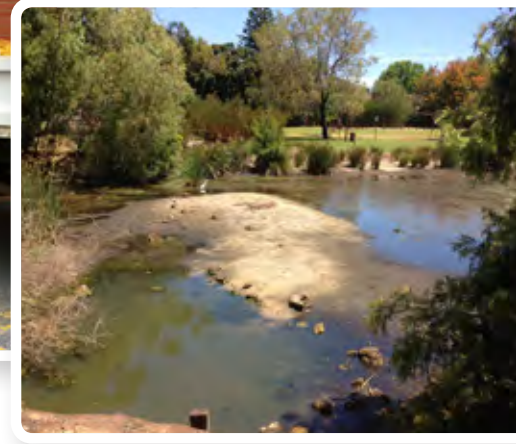
Sediment build-up at Mabel Talbot wetland. Photographer: Giles Pickard, City of Subiaco
