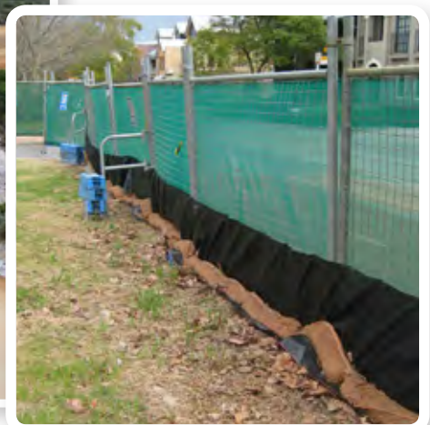
To prevent sediment leaving site, geotextile material should be secured to the site perimeter fence to a minimum height of 600mm. Photographer: Vincent Cusack, The Western Suburbs Regional Organisation of Councils (WESROC)
