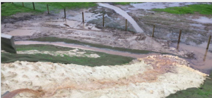
Cumulative impact of sediment contaminated rainwater washing from road to creek at a site that was not fully rehabilitated to control localised erosion
