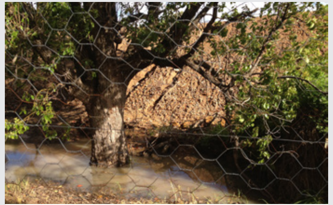
Example of inappropriate separation distances to vegetation and watercourses when infill is brought in
