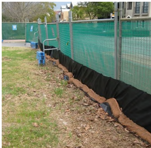
Figure 8: Sediment fencing installed on a development site, designed to capture sediment and prevent it from leaving site. Image source: Bronwyn Scallan, Perth NRM
