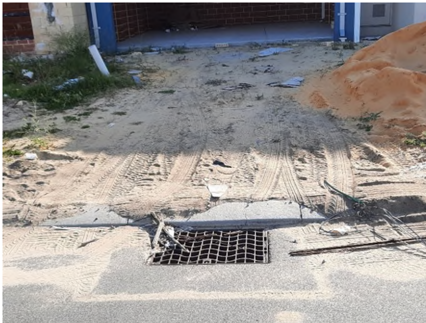
Figure 1: Sediment from a building site entering a drain. Image source: Bronwyn Scallan, Perth NRM
